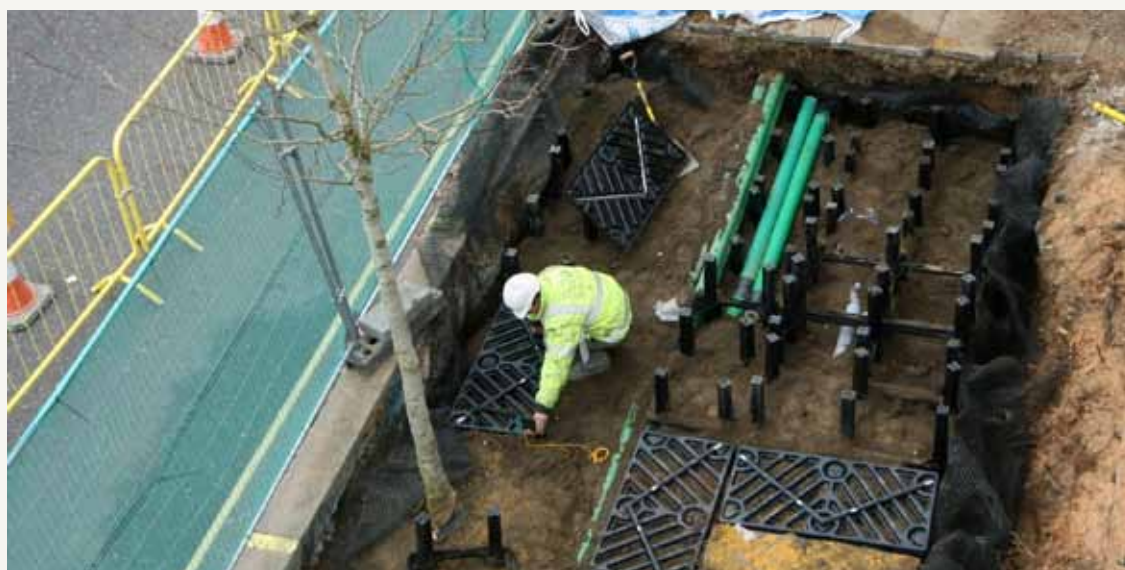
Installation of the 'Silva Cell' modular cell system ensuring new street trees planted in front of the new RAF Bomber Command Memorial in London will grow big. © Jeremy Barrell
